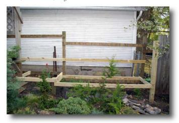
Construction involved first taking down the old fence section that was in need of removal and then building the framework strong enough to hold the weight of potted trees.
